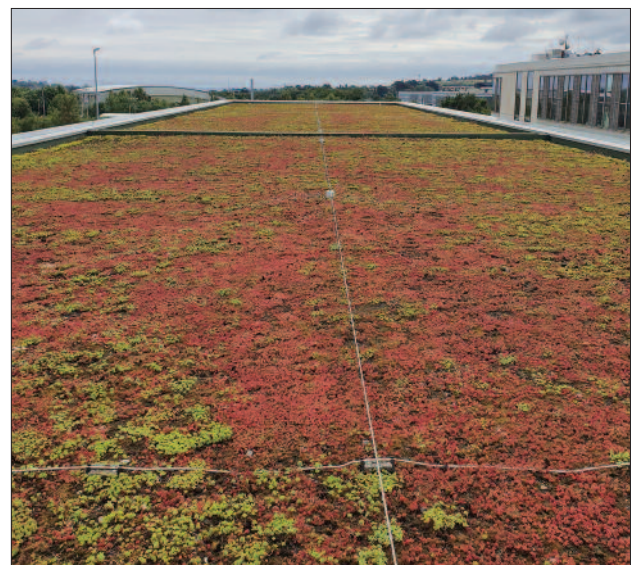
Green roof on Ballyogan depot addressing stormwater runoff
