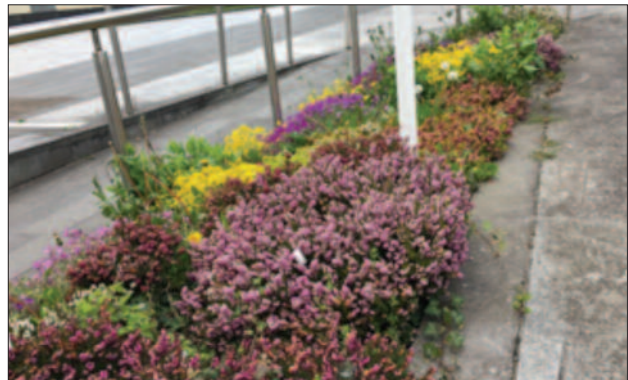
Simply removing Kerbs and correct cambering allows water to attenuate into a mini-raingarden. Combined with other SuDS features, it is that collective and integrated approach that provides for the best surface water management. Clonmel, Co. Tipperary.
